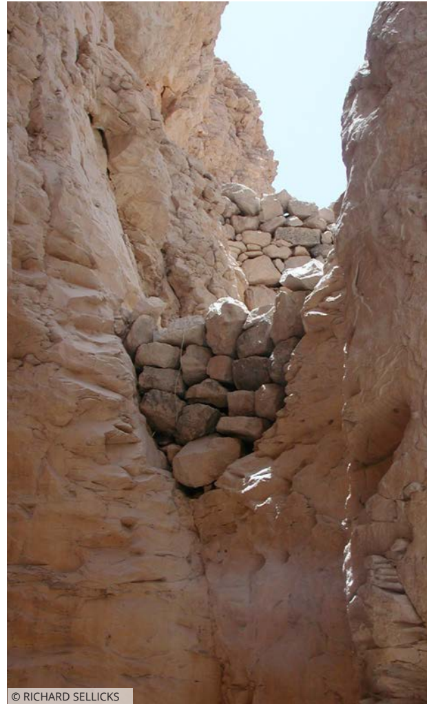
Such a spot is highly vulnerable to floodwaters cascading down from the gully, so a series of dams were built in the watercourse to protect the royal tomb (above). And it worked—Thutmose III's tomb was never flooded.
