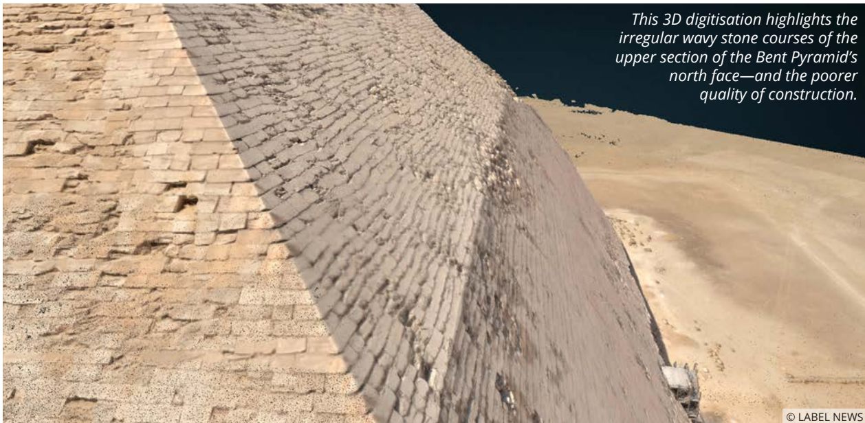
A rush job. The 3D digitisation reveals the wavy courses of the upper part of the north face. These courses are very irregular, using construction blocks of many different sizes and forms—it was finished in hurry.
