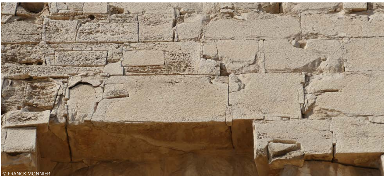
(ABOVE) A detailed look at some of the cut stone repairs, situated a few metres above the ground, on the north face of the Bent Pyramid. A smooth finish was clearly important.
