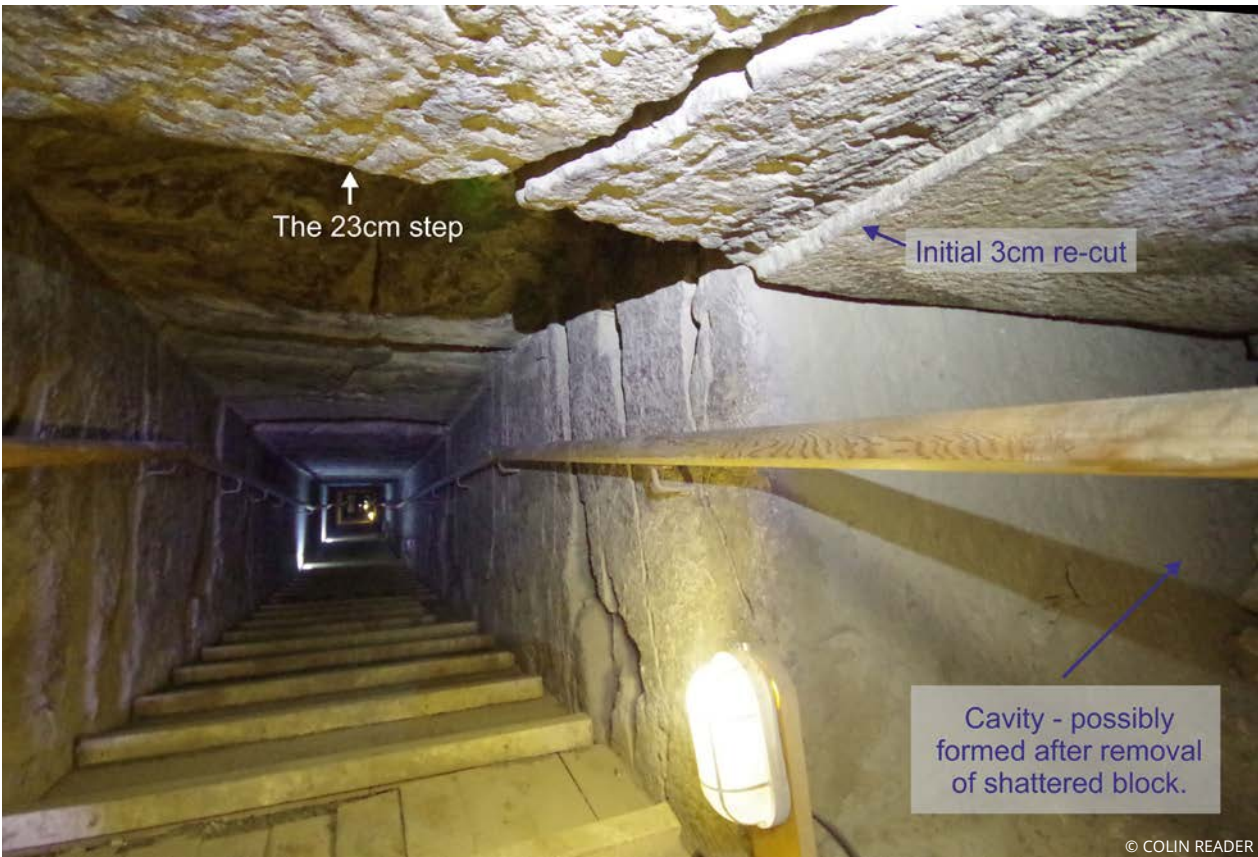
Figure 9. The major dislocation in the Northern Passage, showing the 23 cm step in the ceiling, and (to the right) the
